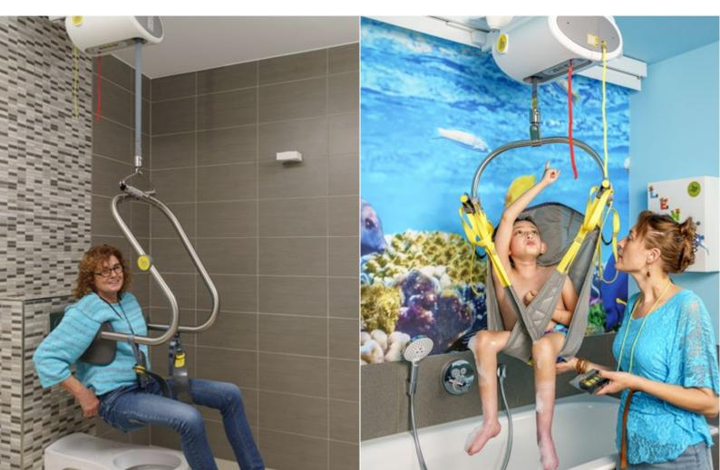
A ceiling track system can connect you between your chair, bed, bath, and toilet to make easy efficient transfers. An authorized SUREHANDS<sup>®</sup> installer will make the necessary modifications to the home so the optimal track design can be provided.
